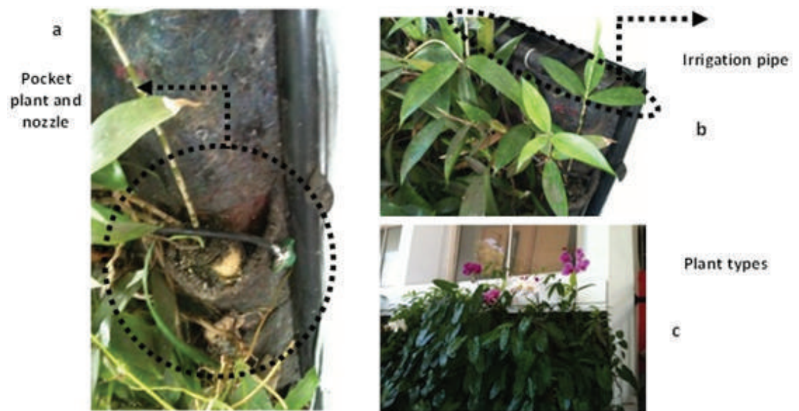
Figure 2: Detail of vertical garden model (a) . Pocket plant and nozzle; (b) . Irrigation pipe; (c) . Types of the plant in the vertical garden model [16].
